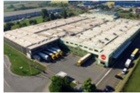
Corrugated board plant Budapest (H)
