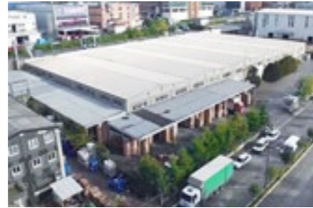
Corrugated board plant Istanbul (TR)
