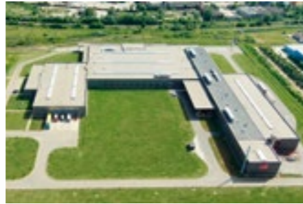
Corrugated board plant Târgoviste (RO)
