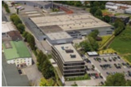
Corrugated board plant Frastanz (A)
